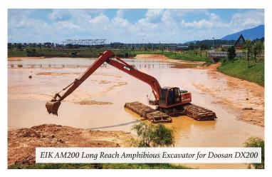
access deeply settled pockets of silt and reshape selected areas of the pond to improve water distribution. As clearing progressed, the pond gradually regained depth and restored more consistent flow during rainfall.
