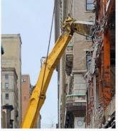
Fully modular in design, the joints are fitted with hydraulicoperated pins. Assembly and disassembly becomes a breeze, saving time, cost and manpower. One best appreciates the convenience of the hydraulic pins especially when carrying demolition works in busy town areas. Every minute saved on assembly and disassembly translates into productivity gains for the many who have to put up with disruption to their routine.
